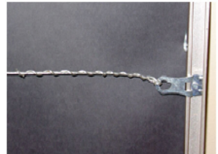
Secure lead through ring tightly wound
