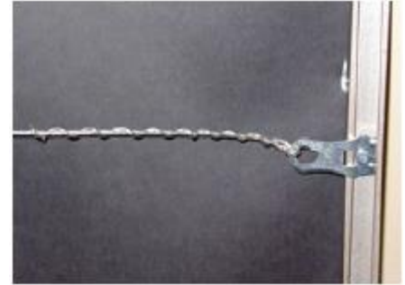
Secure lead through ring tightly wound
